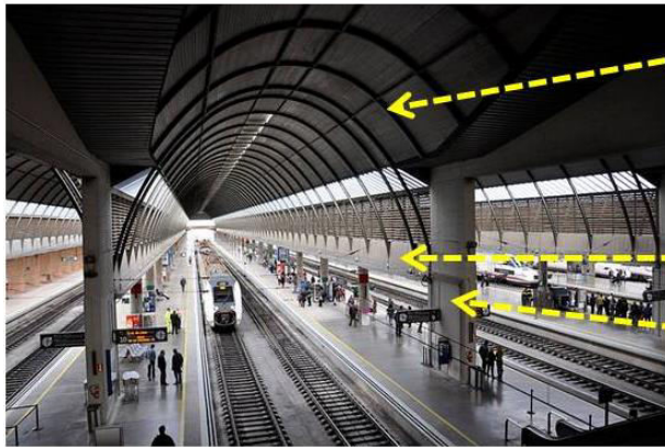
Figure 14 Santa Justa Train Station, Seville, Spain
