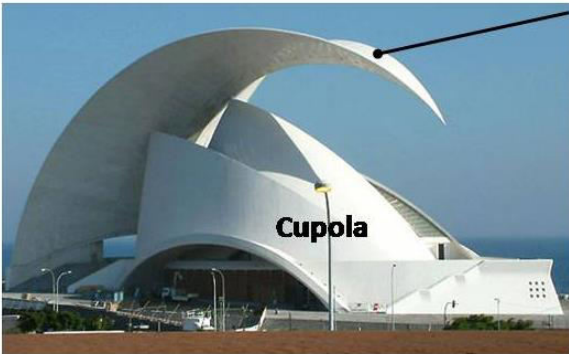
Free Standing Shell Roof covered with ceramic tiles
