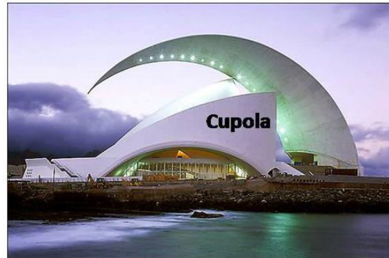
Free Standing Shell Roof covered with ceramic tiles
