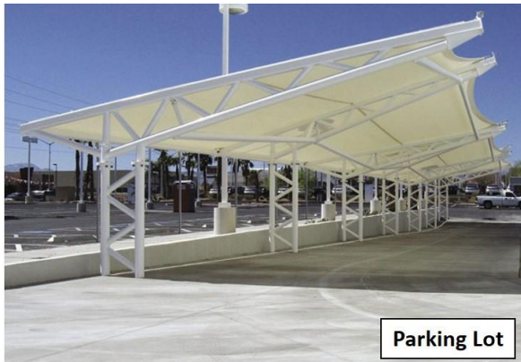
In between two steel tubular truss stretched membrane roofing
