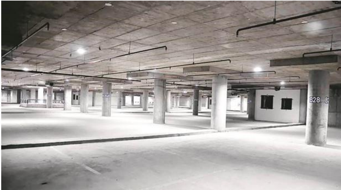
Figure 13 : Multi-level car parking at Chandigarh, with drop panels
