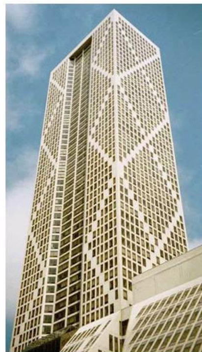
Onterie Center (1986), Chicago, 174 m ,58 stories
