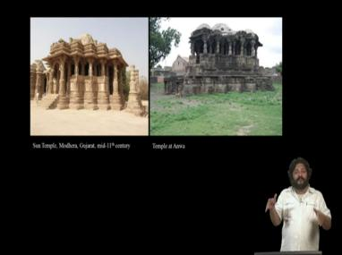
And the plan is semi-open which means you only have walls still about waist height, above which the whole sabhamandapa, the space in front of the sanctum is enclosed by pillars, half pillars above which is the roof in the form of corbel domes.
