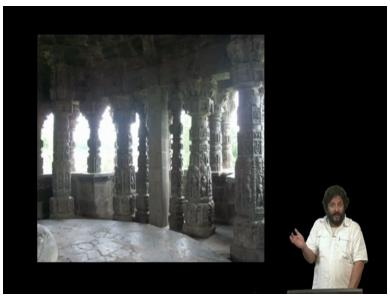
As though this picture was not enough, here you can really see it. Ignore the concrete block support that was put in by the archaeological survey of India to ensure the structural stability. But what you see here is two wide columns with a beam on top, the beam has very obviously cracked. Because it was cracked, the archaeological survey put in a column of concrete blocks.
