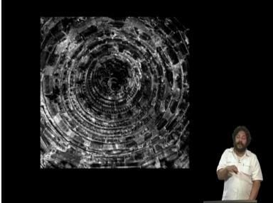
The dome, as we mentioned on the inside of the sabhamandapa, is corbelled, which means it is not built out of true goose bar stones but it is built by successively moving each course of stones slightly further till they meet right at top. This is a technique you find in the sabhamandapas of almost all giant temples in this period.
