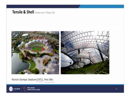
So, tensile structures one of the famous architect was Frei Otto, so this is the Munich Olympic stadium; which is designed in the 1972 by Frei Otto. So if you look at this has a series of steel mim; steel mast which is holding this roof form of this on the gallery so gallery with a this tensile members. So these are the tensile members you can see in this photograph which is on top of this gallery.
