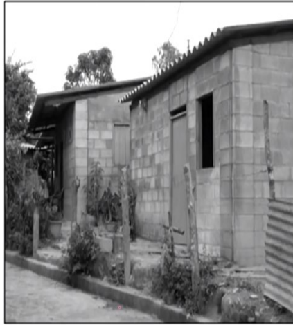
Figure 12.5 Houses that have been simply finished in Hacienda Nuevo Oriente, five years later
