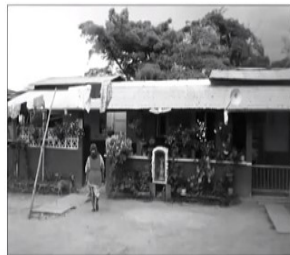
Figure 4.2 Repaired houses Residents acquired loans and subsidies and built the type of house they wanted according to their needs, capacity to work in construction and availability of their own resources
