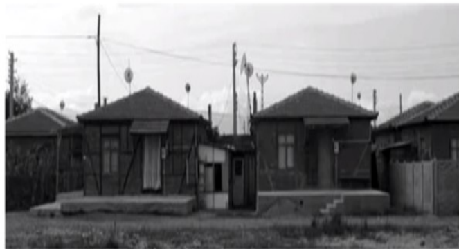
Figure 11.5 UMCOR settlement completed
