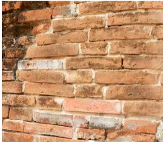
In the new brick laying work there is a lot of room for improvement
