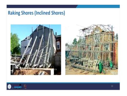
This is another one where you can see that how like in this place it is only the iron, like your steel tube being used and here it is instead of that, the you know the thrust being used to support it, with your horizontal member and inclined shores and this is another one where it is also supporting a wall.
