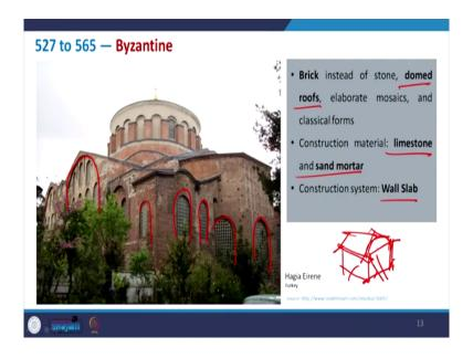
Now, come to the Byzantine where like stone is being replaced with some brick instead of stone and then dome roof like in even in Pantheon in Rome we have seen that. So, it is being used and here along with that you can see that you know arch use of arches in for the window being used, even for the structure these huge you know the roof. So, again the pitch roof has come into the picture and construction material basically limestone and sand mortar and construction system is wall slab.
