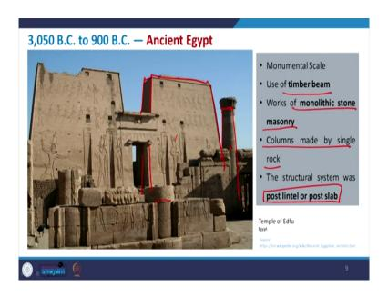
Not only pyramid even that period in Egypt they have also constructed other structure where they have used the timber beam and then this is monolithic stone masonry. So, you can get this particular wall. So, a piece of you know stone they are they have used, then the columns made by single rock.
