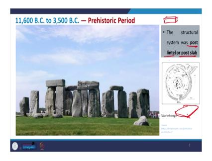
So, this is again pre historic example and this is the Stonehenge following the same you know same kind of arrangement of structure post lintel or post slab. So, depending on the span or the area of the stone we used either we call it slab when it has a considerable you know area, length and width, and when it is just you know just like a piece of like beam so, then we go for this post lintel structure.
