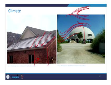
So, here if you see this example here it is a pitch roof made of the concrete tiles. And in this the purpose to make it like with this, like again we go for this you know heavy wall or the cavity wall, so that can maintain the temperature, but along with that the slope will also help to you know you know runoff the snow when it is melted due to the you know sunlight or heat and this is to be used in the rainy areas.
