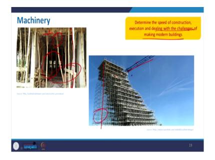
Then the missionary plays an important role. It will determine the speed of construction, then execution and detailing dealing with the challenges of making modern buildings. So, earlier like for the low cost construction or earlier people used to you know have this you know wood baton and then the bamboo as a props to support the structure.
