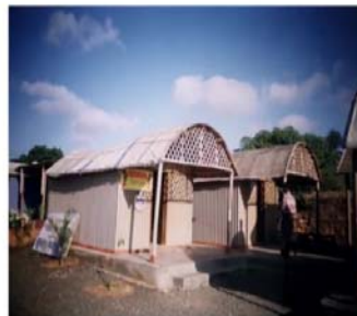
Temporary office made of laminated paper pipes Cost- Rs. 27000/-
