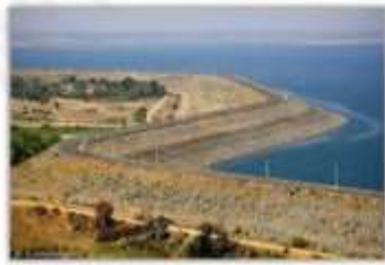
Kangsabati Dam/Reservoir Mukutmanipur, Bankura, West Bengal
